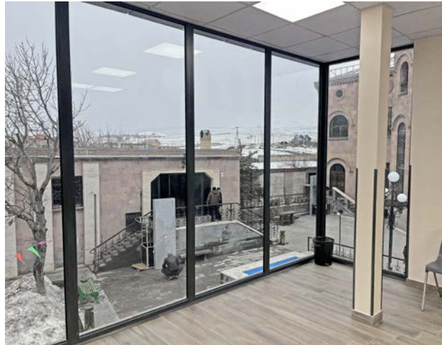
Work on the new rehabilitation center is proceeding apace. csi
